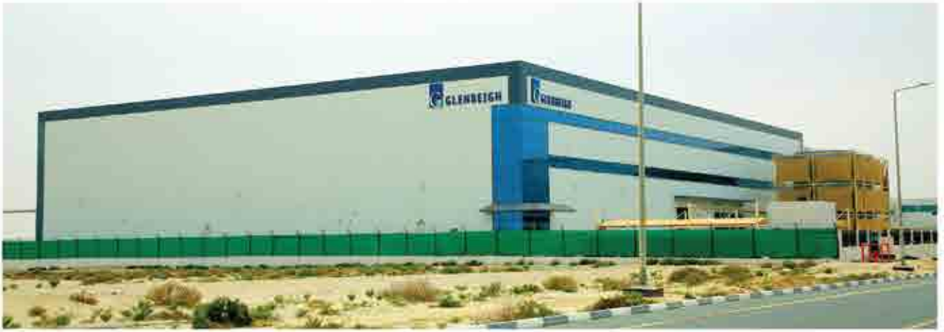
Client : M/S. AL AVON CONTRACTING LLC Project : GLENBEIGH
