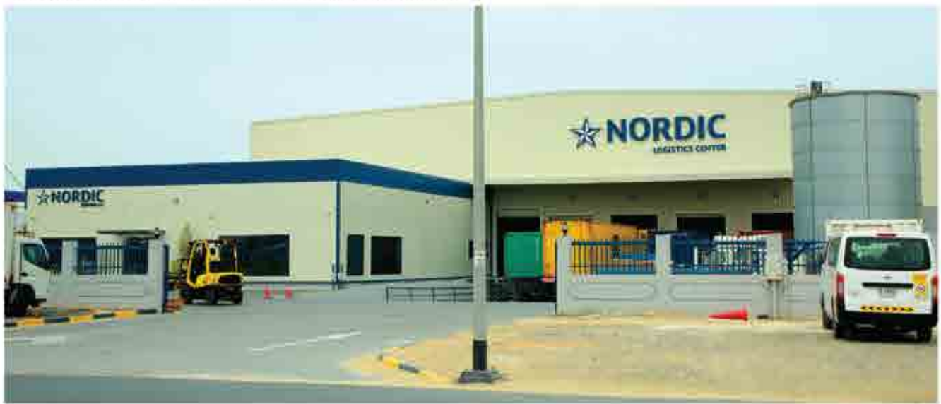
Client : M/S. PENTA EMIRATES CONTRACTING LLC Project : NORDIC LOGISTICS CENTER
