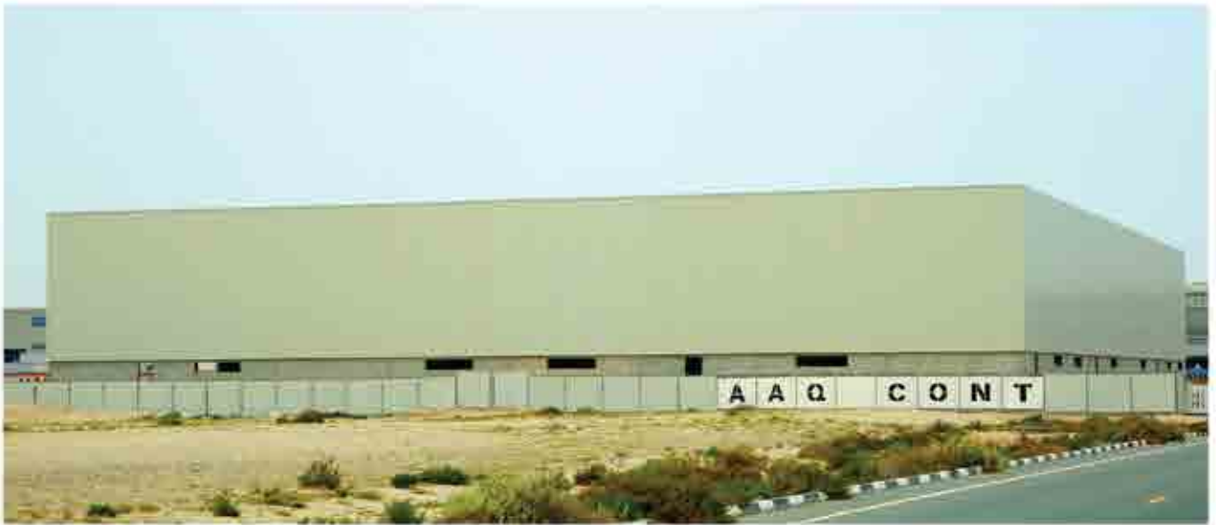
Client : M/S. AAQ CONTRACTING LLC Project : HARMONY LOGISTICS
