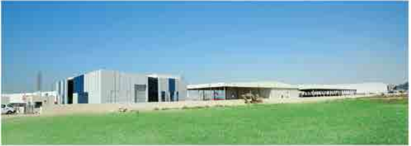
Client : M/S. SPACE MAX CONTRACTING Project : DSS STEEL
