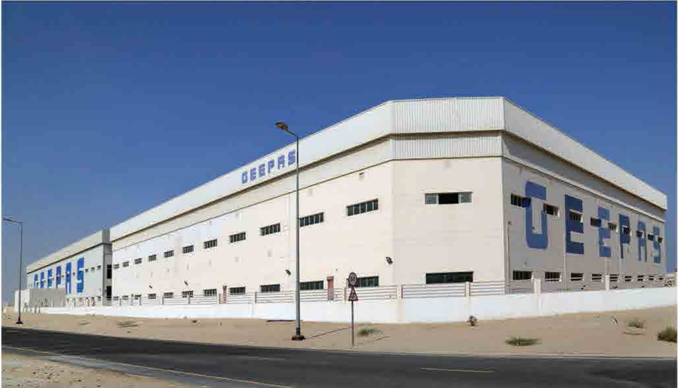
Project: Geepas Client: Al Avon Contracting
