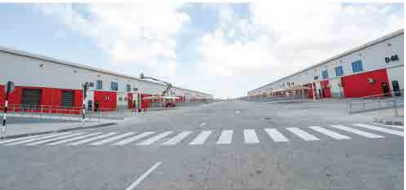
Client : M/S. AMANA CONTRACTING AND STEEL BUILDING CO. WLL Project : PROPOSED WAREHOUSE IN KIZED LOGISTICS PARK
