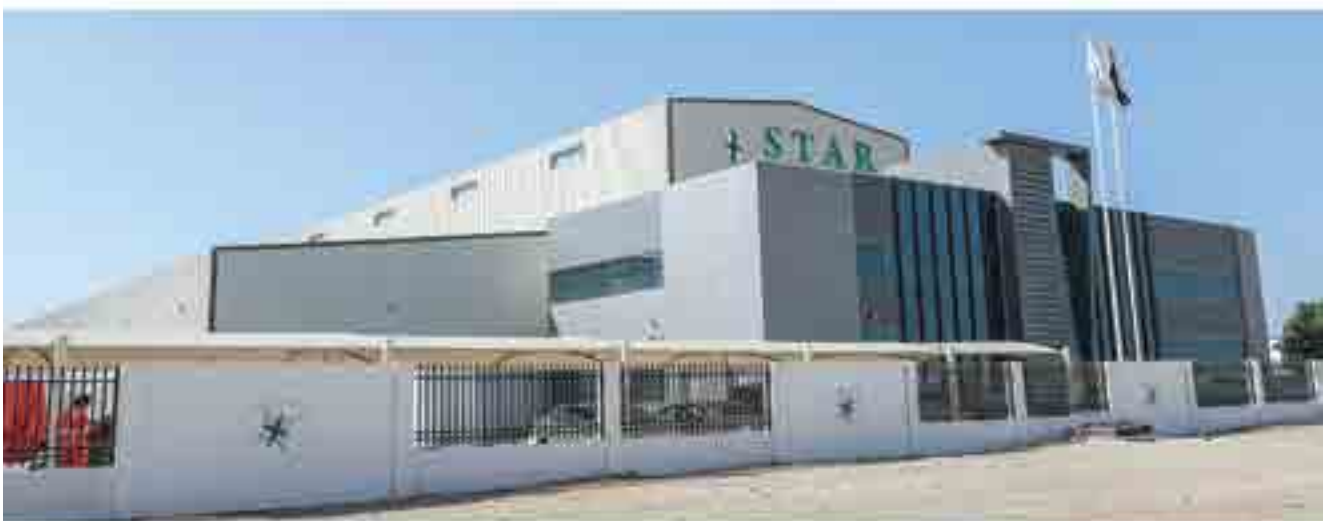
Client : M/S. BRONZE STAR STEEL BUILDING AND CONTRACTING LLC Project : STAR PAPER MILL
