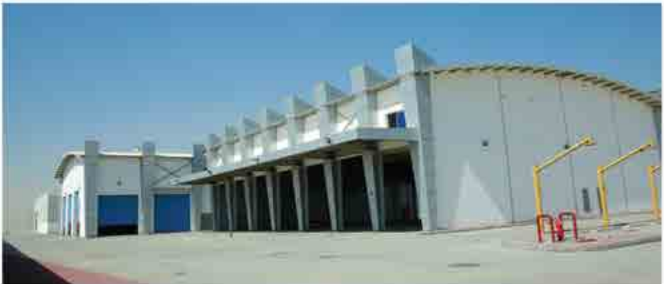
Client : M/S. AL AMAARA CONTRACTING Project : SERVICE BAY BUILDING
