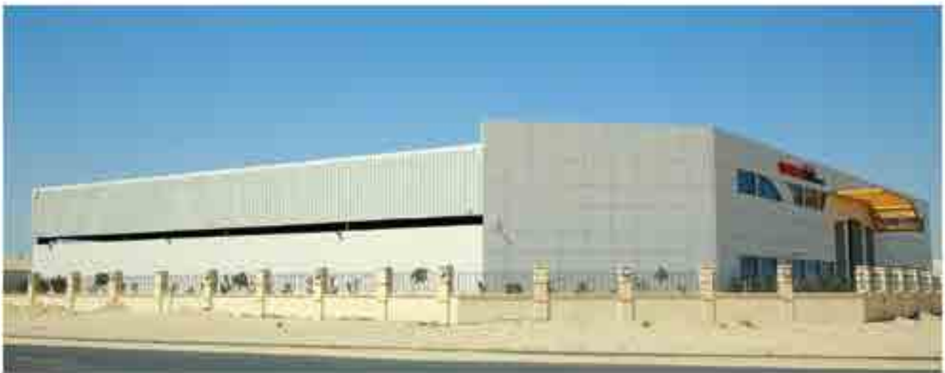
Client : M/S. CLASSIC BUILDING CONTRACTING Project : SUPREME STEEL LLC
