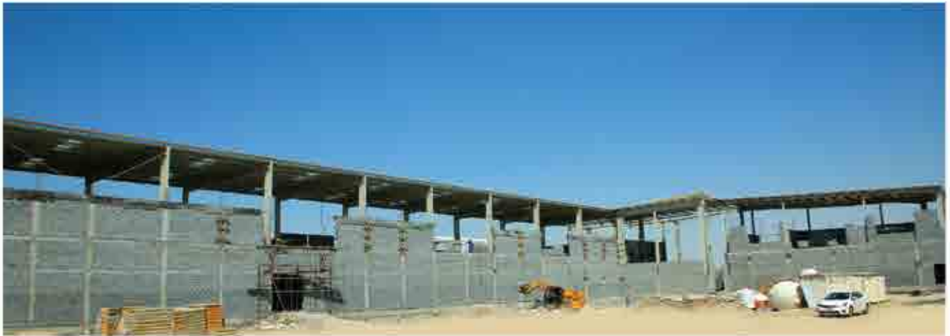
Client : M/S. AL YAZAN CONTRACTING LLC Project : LFI FOOD INDUSTRIES
