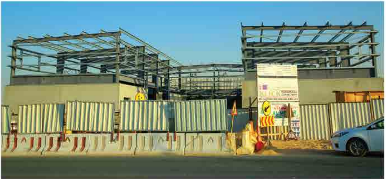
Client : M/S. AL MEHAR CONTRACTING LLC Project : WAREHOUSE (G+M)
