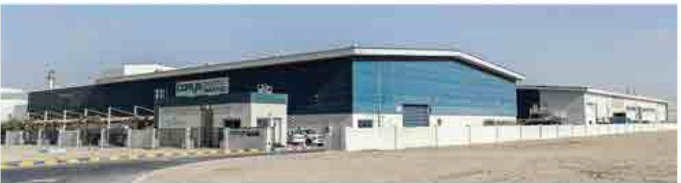
Client : M/S. PROMPT STEEL BUILDING AND CONTRACTING Project : CORYS'S PLASTIC INDUSTRIES
