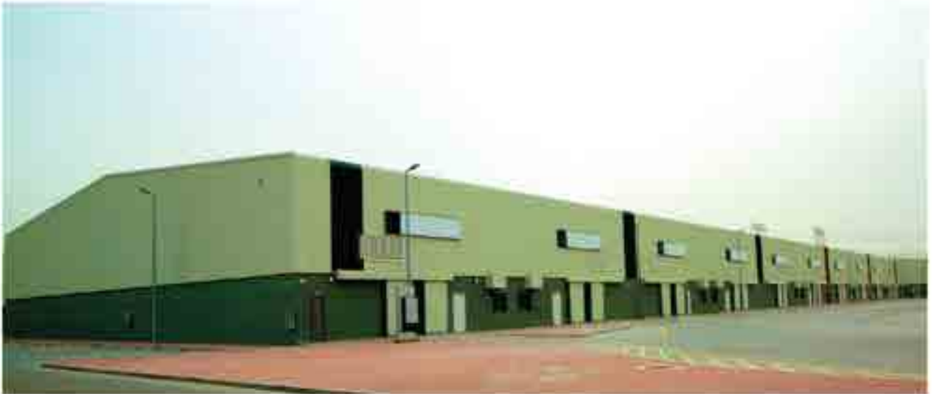
Client : M/S. RAQ CONTRACTING LLC Project : ETJAR INVESTMENT LLC
