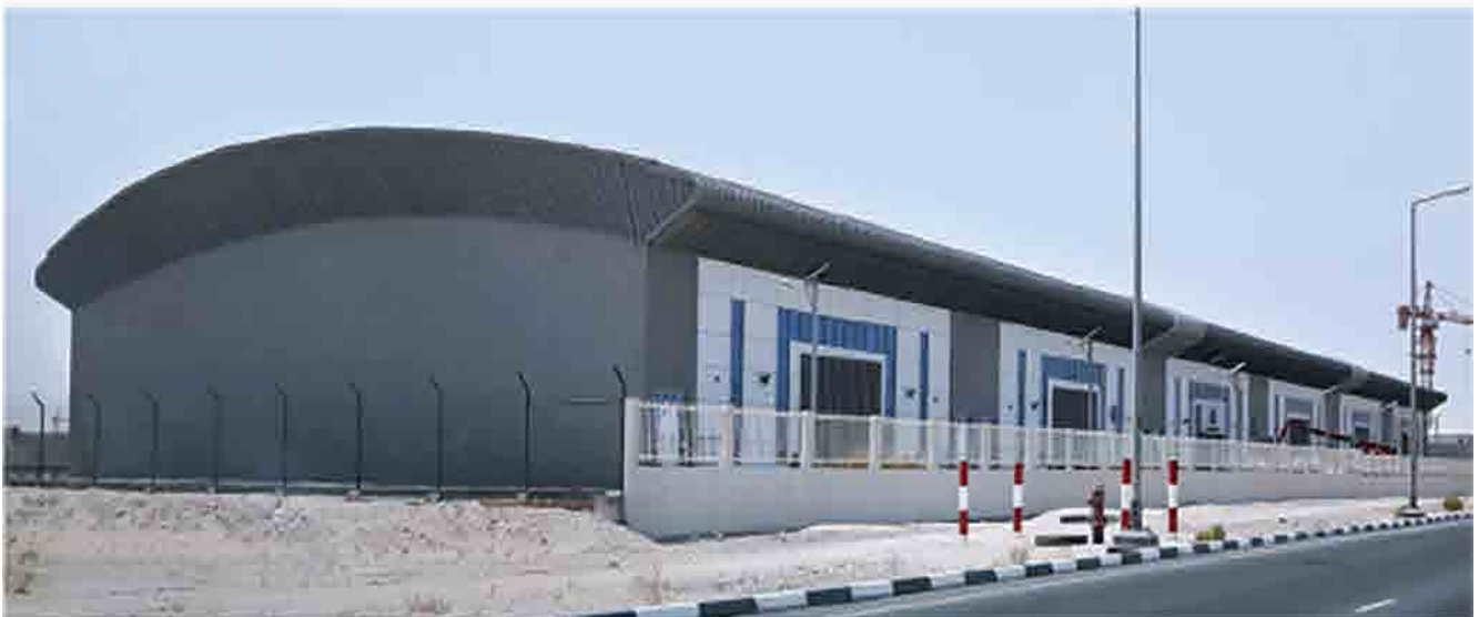
Project: Aero Space Supply Chain Client: City Diamond Contracting LLC
