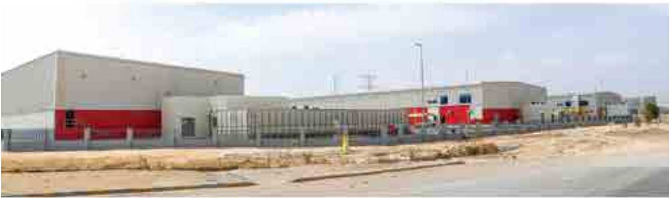
Client : M/S. AMANA CONTRACTING AND STEEL BUILDING CO. WLL Project : PROPOSED WAREHOUSE IN KIZAD LOGISTICS PARK
