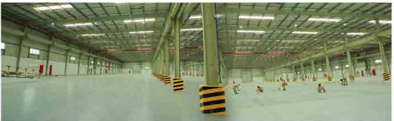
Client : NAFFCO (PENTA EMIRATES)
