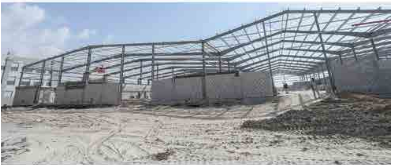
Client : M/S. DHAFIR TECHNOLOGIES LLC Project : PROPOSED COATING SHELTER
