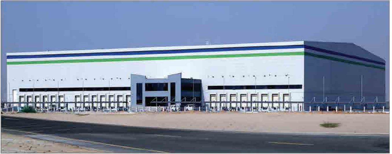
Project: Global Shipping Client: City Diamond Contracting
