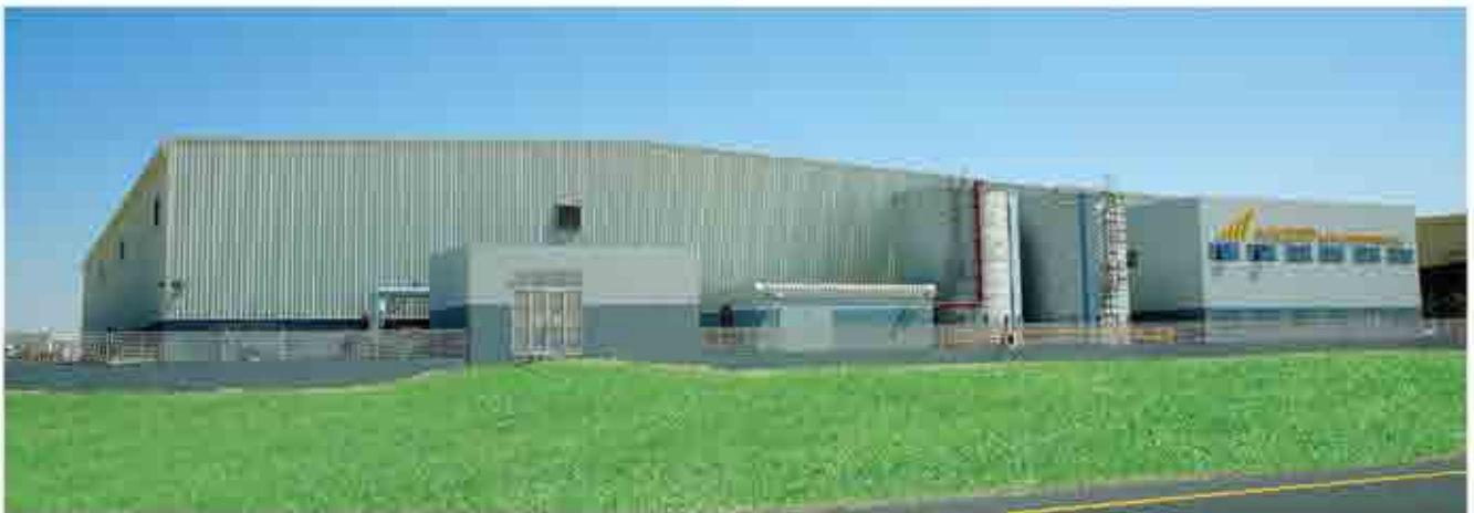
Project : M/S. ASCEND METAL INDUSTRIES
