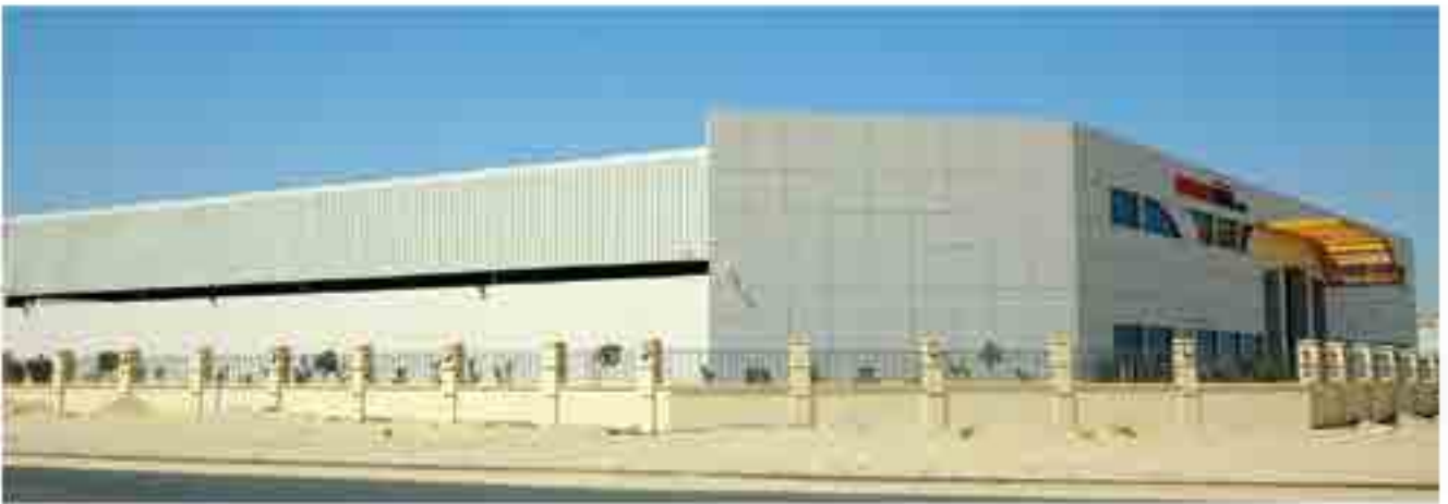
Client : M/S. LOYAL BUILDING CONTRACTING Project : SEVENSEAS STEEL INDUSTRIES LLC
