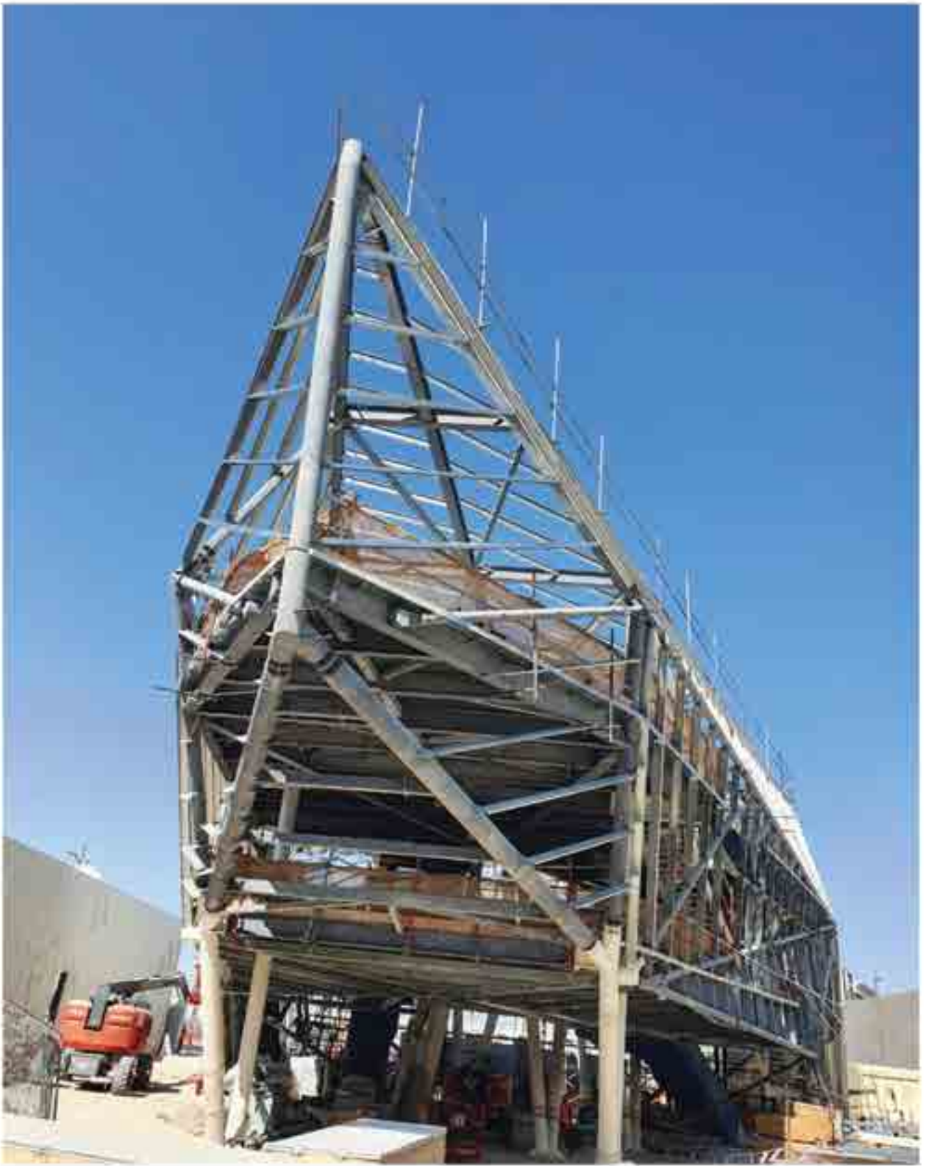
Client : M/S. SAM BUILDING CONTRACTING Project : SERBIA PAVILION (EXPO DUBAI)
