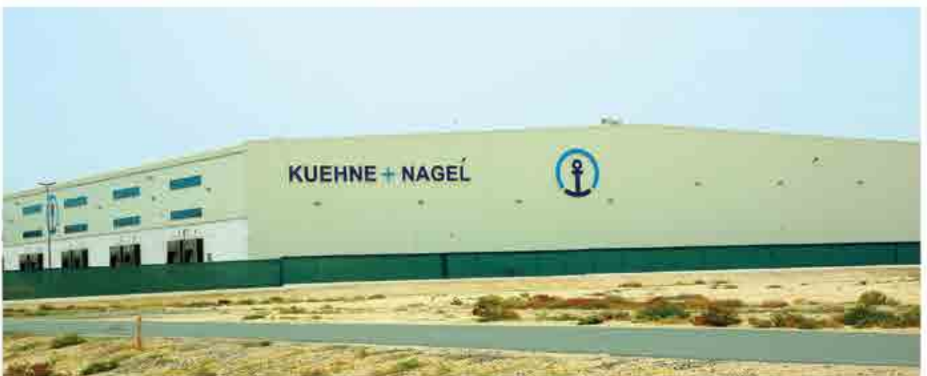
Client : M/S. AL AVON CONTRACTING LLC Project : KUEHNE + NAGEL
