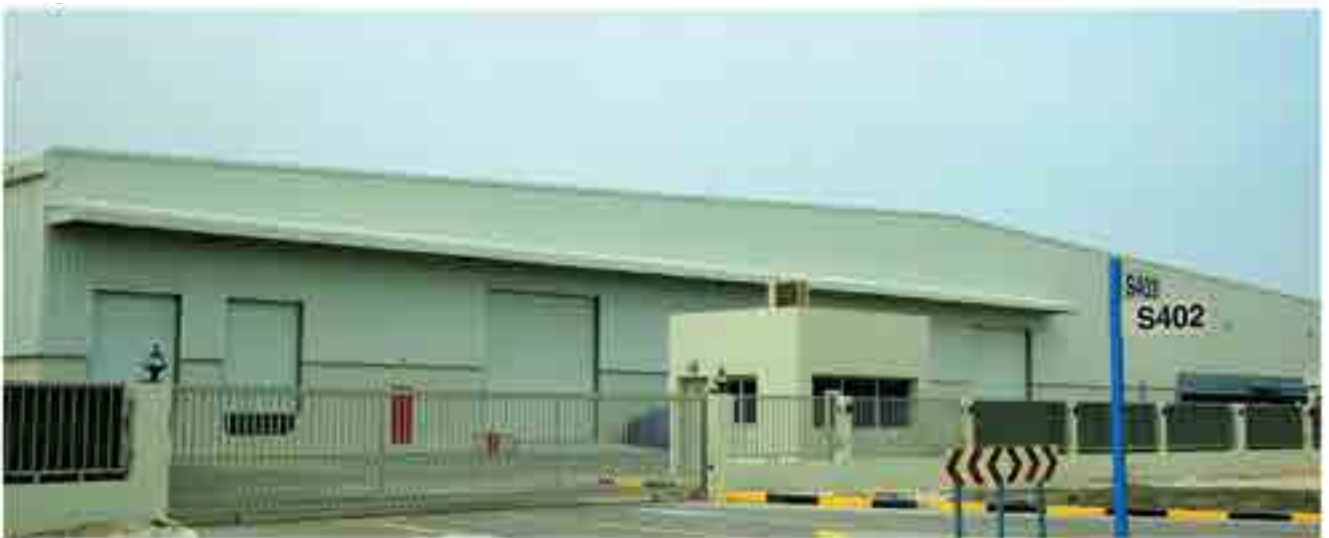
Client : M/S. AL AVON CONTRACTING LLC Project : ACCESS WORLD LOGISTICS
