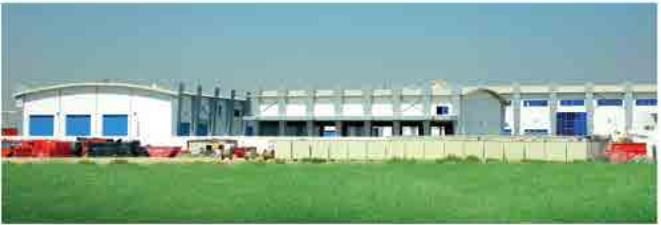
Client : M/S. AL AMAARA CONTRACTING Project : SERVICE BAY BUILDING
