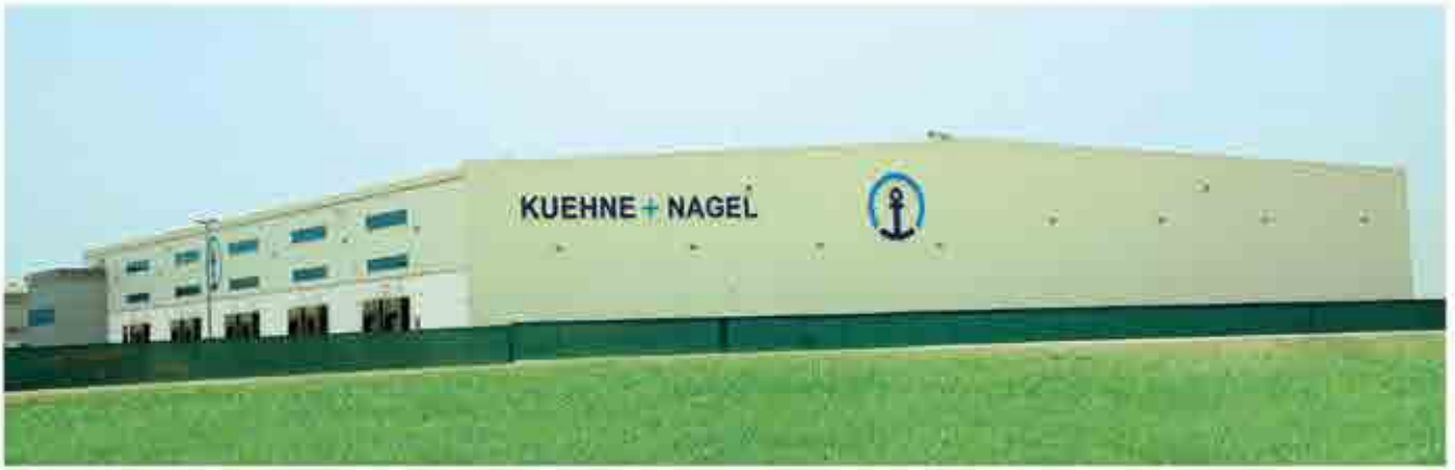
Client : M/S. AL AVON CONTRACTING Project : KUEHNE + NAGEL WAREHOUSE
