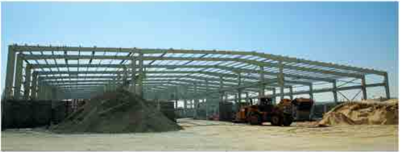
Client : M/S. MODULAR CONCEPTS LLC Project : WAREHOUSE & OFFICE
