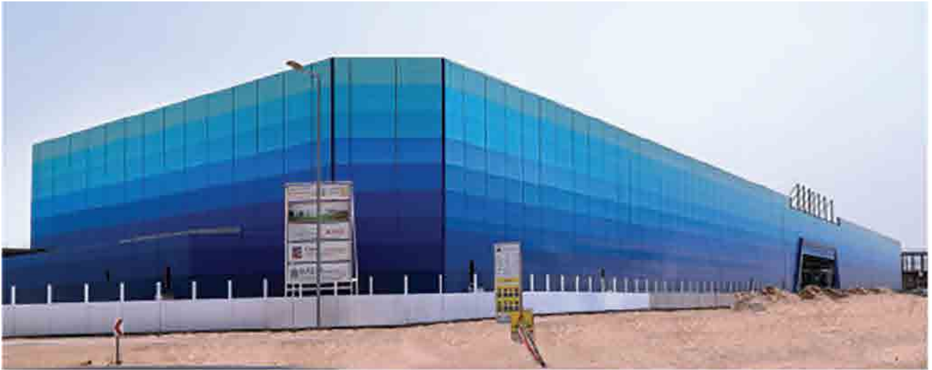
Project: Nesto Client: Ranicon Contracting
